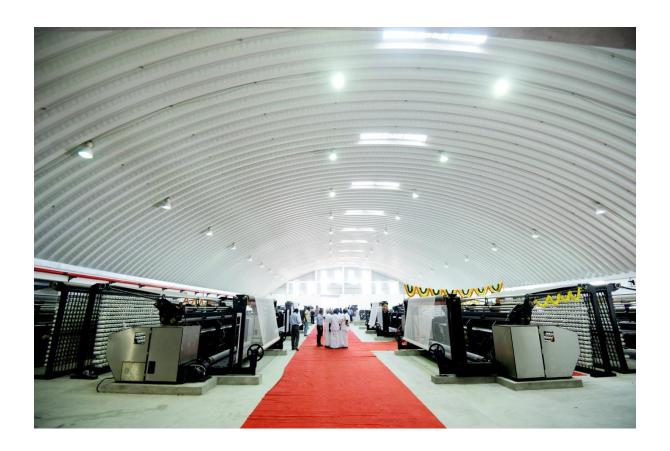
The fishnet factory building was built with technical consultancy with M/S KITCO (Kerala Industrial and technical Consultancy Organisation), Govt undertaking. This has helped us to use the truss less technology for factory shed of dimension 36m x 60m without any pillar. This is the first time this technology has used in Kerala for construction of any building of factory shed. The service of the consultant was useful in timely completion of the project.
